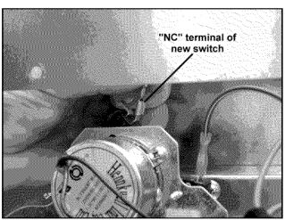
13. Disconnect the wire from the fan to the 170° thermostat. Connect this wire to the piggyback terminal on the #3 (318052585 – Red) wire. Connect these two wires onto the open terminal of the 170° thermostat.
